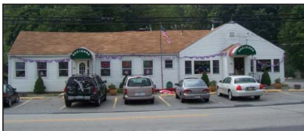
Existing restaurant on Route 218 lacks a landscaped buffer
