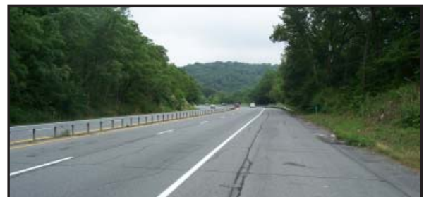
Route 9W, looking south
