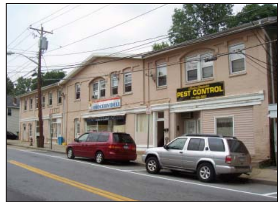
A building in need of sign improvements
