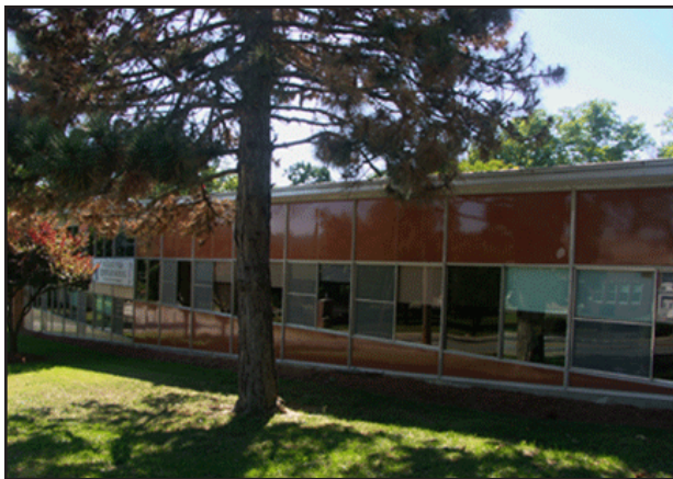
The Highland Falls Elementary School
